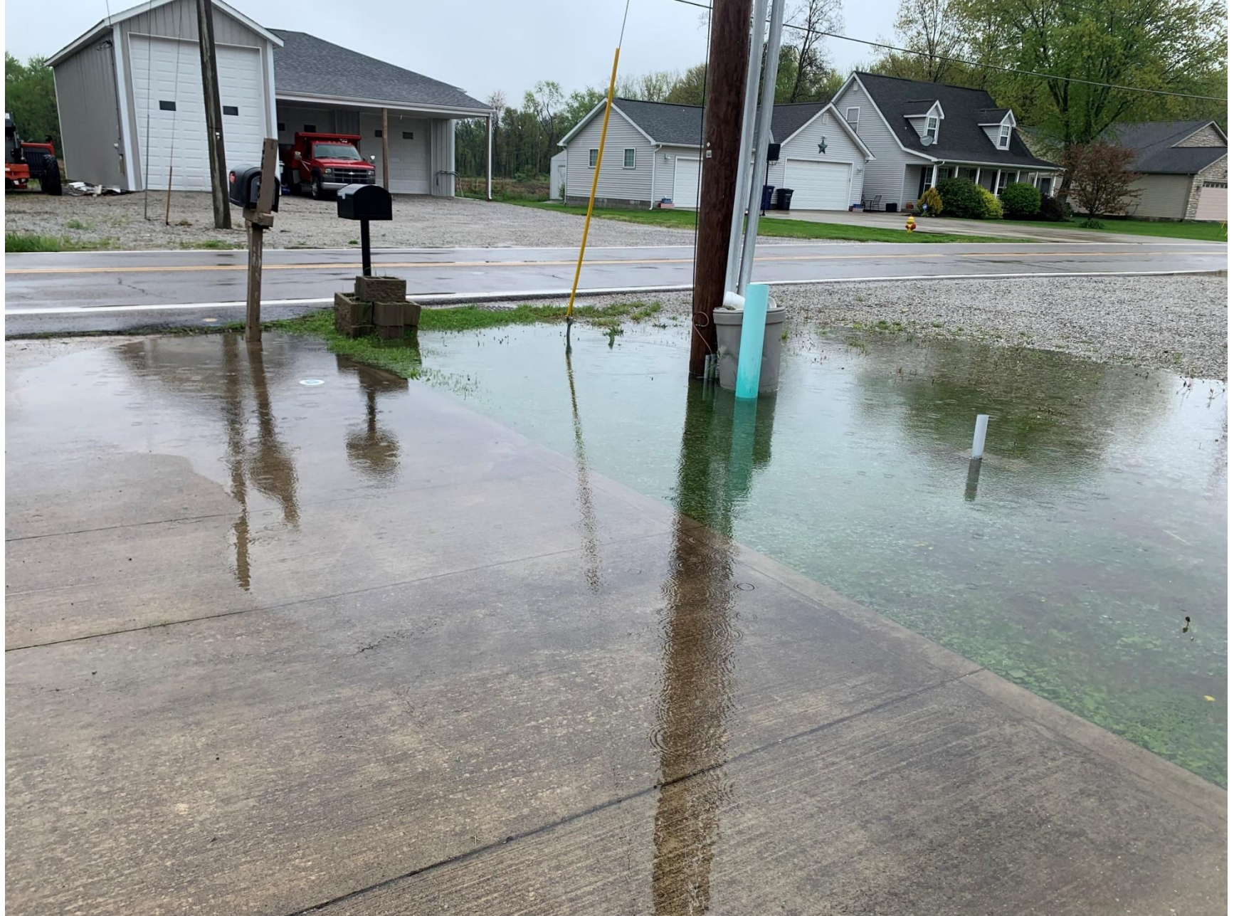
Typical Flooding 3685 North Bank Road South Side Looking North
